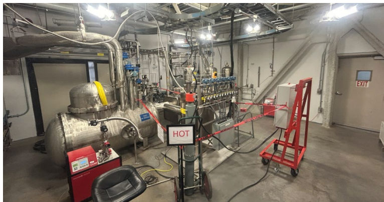
Figure 6. New CMS Oil Processor (a) and Existing CHL Oil Processor (b)
