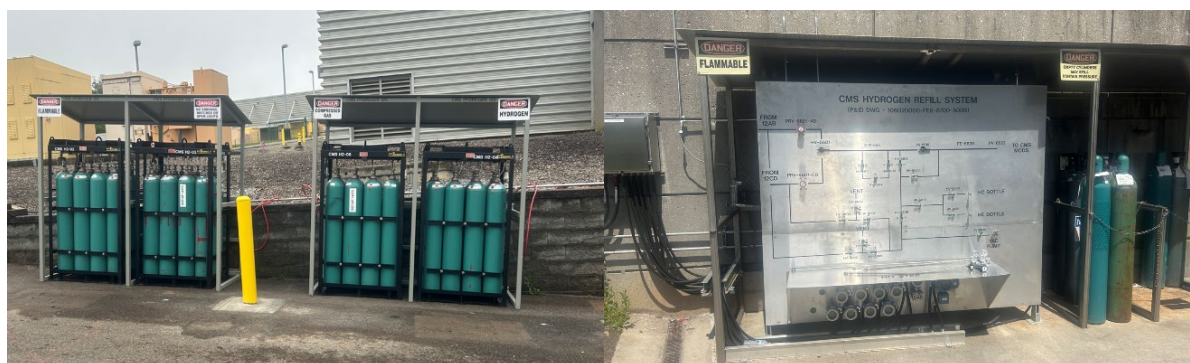
Figure 8. Hydrogen Refill System (a) Gas Supply Stations (b) Instrumentation & Control Panel
